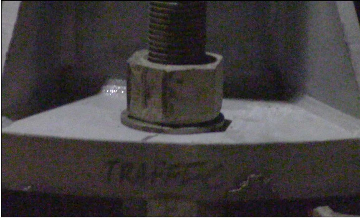
Figure 1.29 - Post Tightening with Reference Marks Shown
