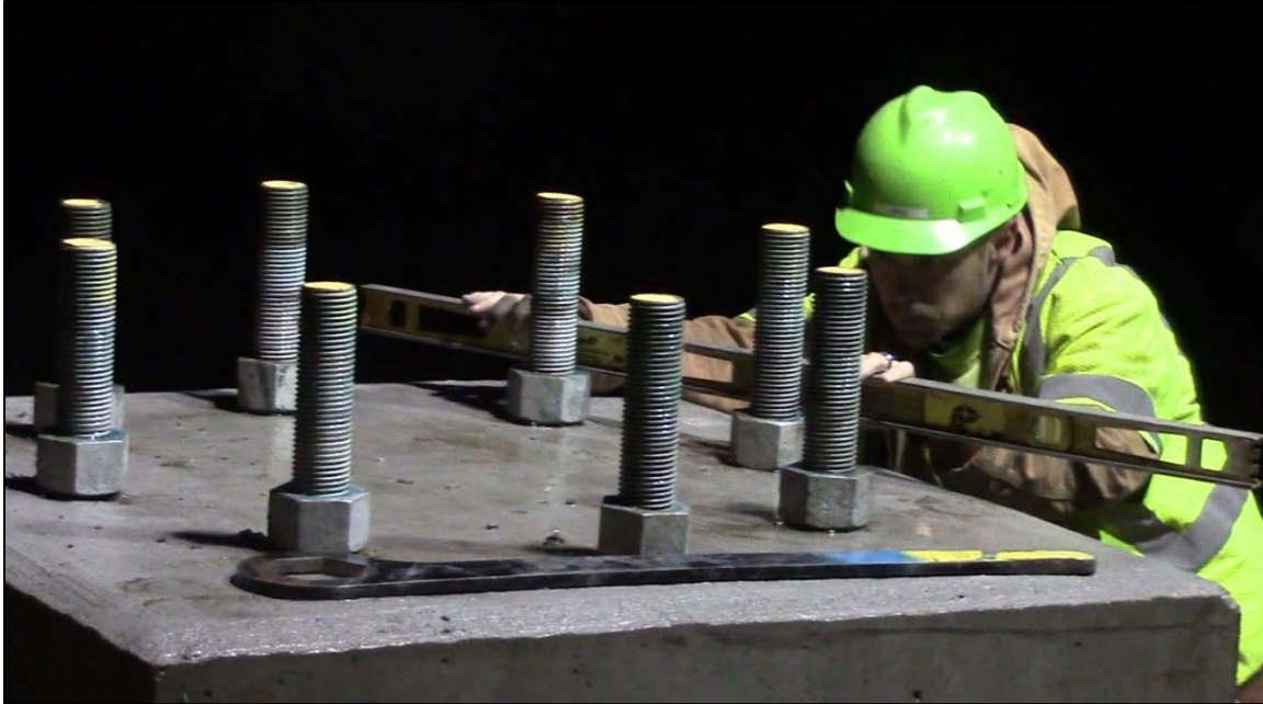
Figure 1.23 - Leveling During Iowa Site Visit
