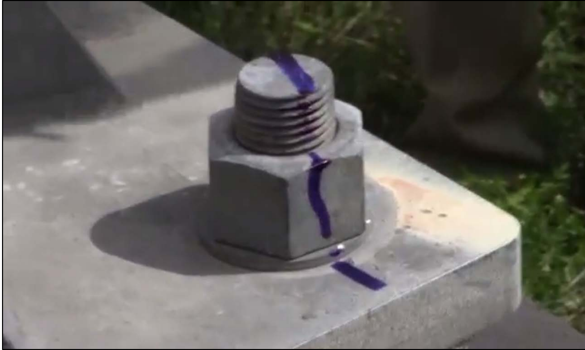
Figure 1.19 - Reference Marks Used During Maintenance
