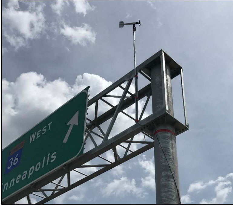
Figure 3.10 - Anemometer Placement
