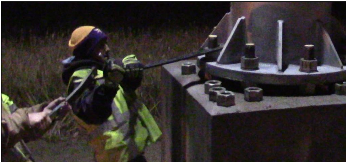
Figure 1.28 - Final Tightening After Making Reference Marks
