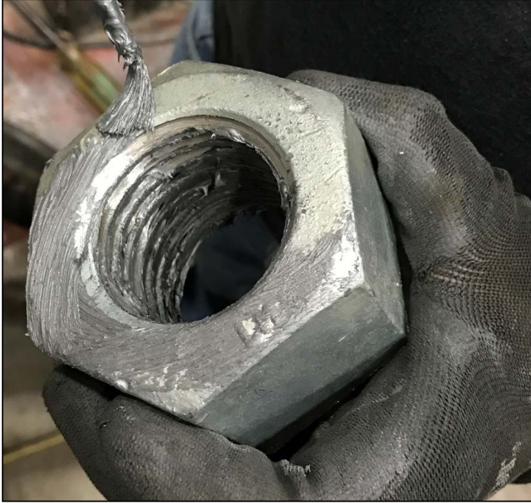
Figure 2.4 - Lubrication of Nut Bearing Surface
