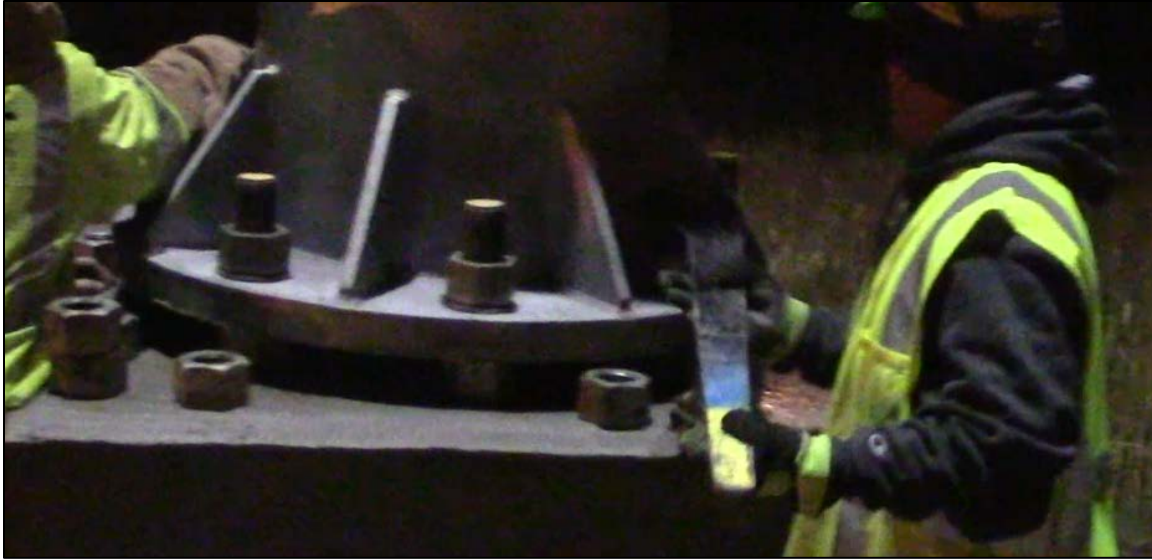
Figure 1.27 – Snug-tightening of Bolts
