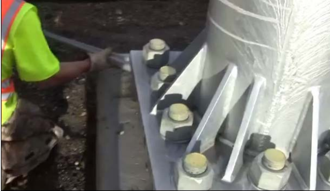
Figure 1.13 - Leveling Nut Tightening in Minnesota
