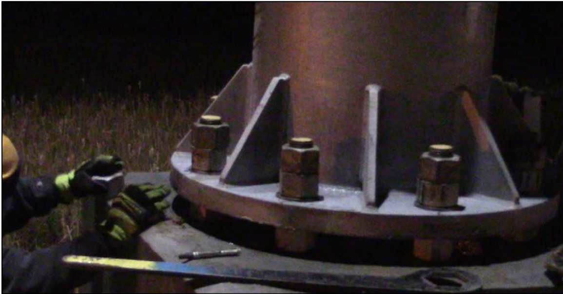
Figure 1.30 - Final Assembly with Jam Nuts
