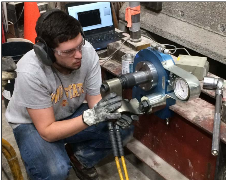
Figure 2.1 - Hydraulic Wrench Tightening
