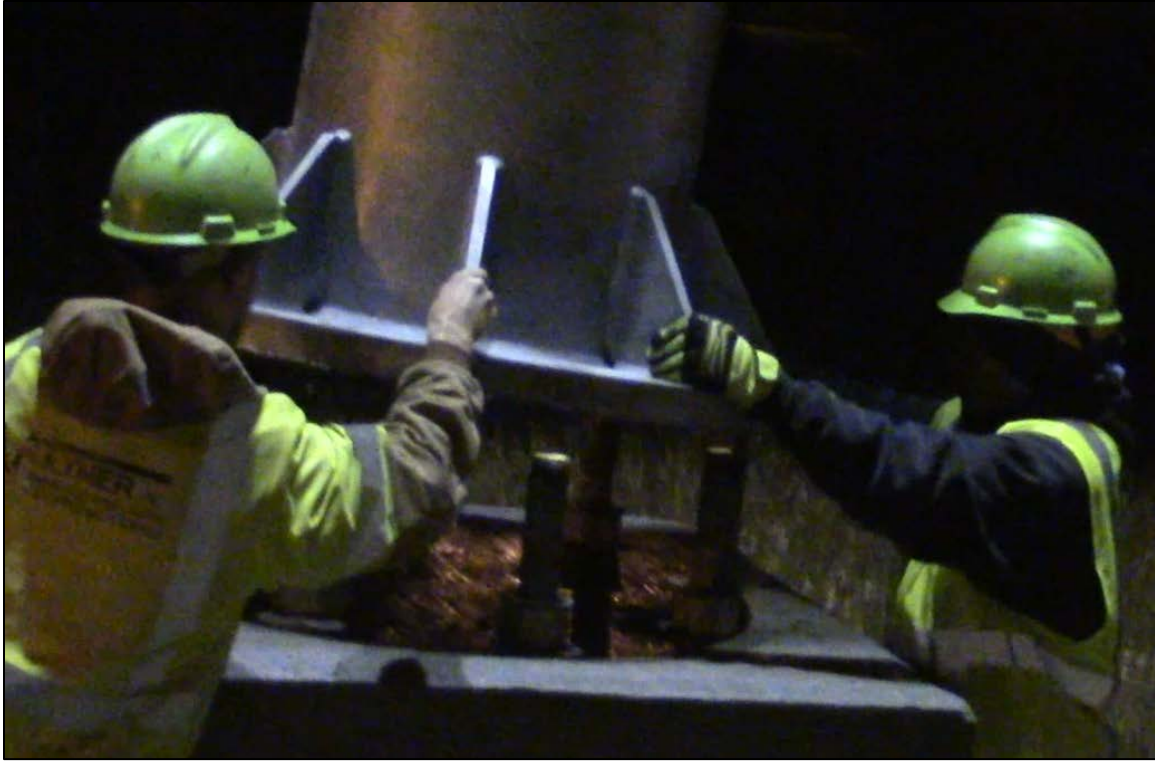
Figure 1.25 - Installation of Pole
