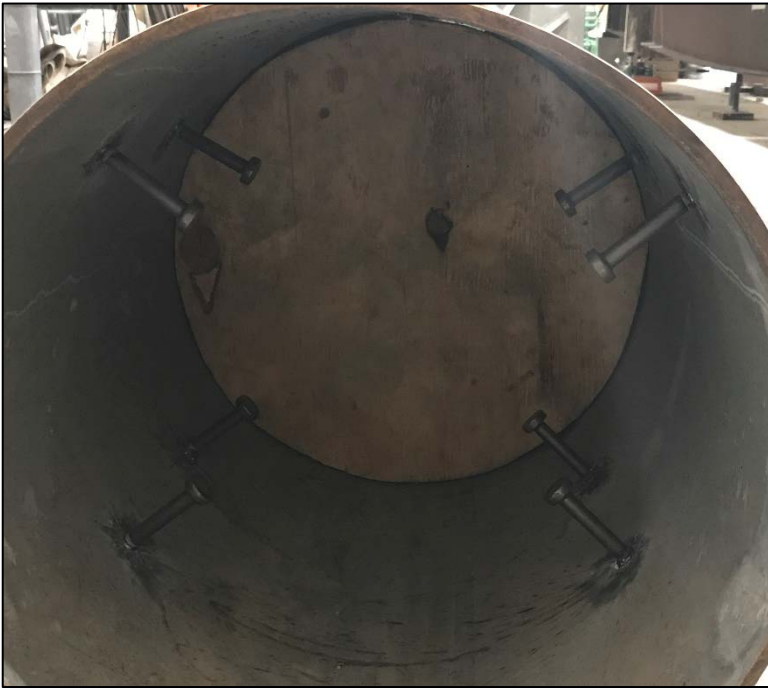
Figure 3.31 - Shear Studs and Wood Form Inside Sign Post
