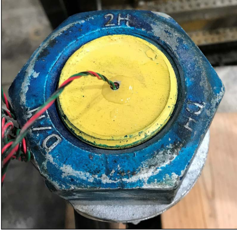
Figure 3.6 - Anchor Bolts after Strain Gage Installation
