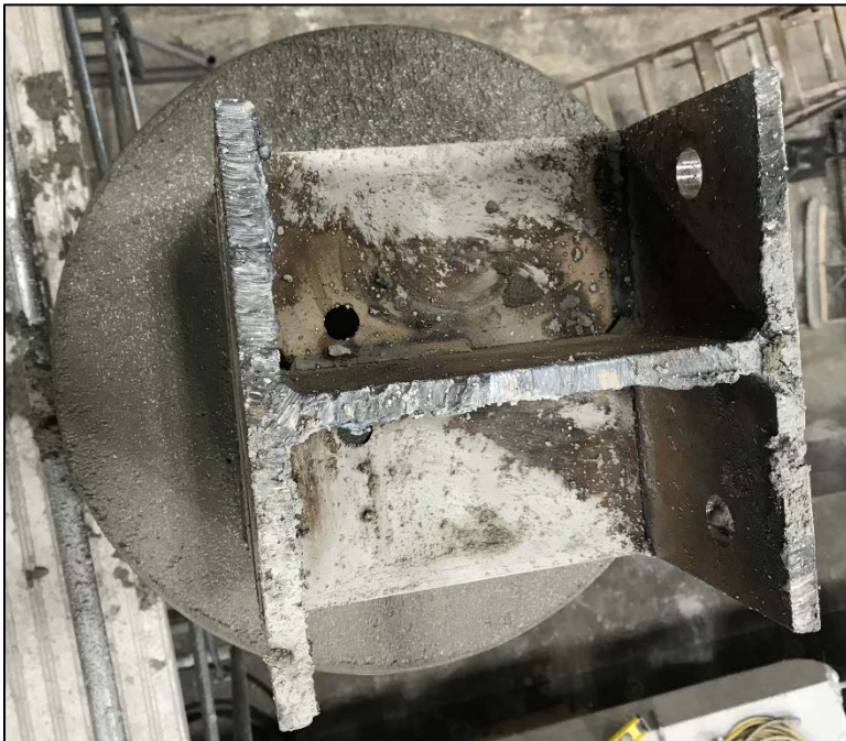
Figure 3.35 - Top View HP10x57 Curing in Concrete
