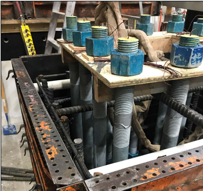
Figure 3.29 - Rebar, Anchors, and PVC Placed in Formwork
