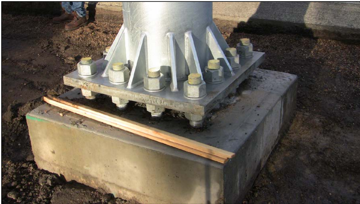
Figure 1.10 - Overhead Truss Baseplate and Anchor Bolts
