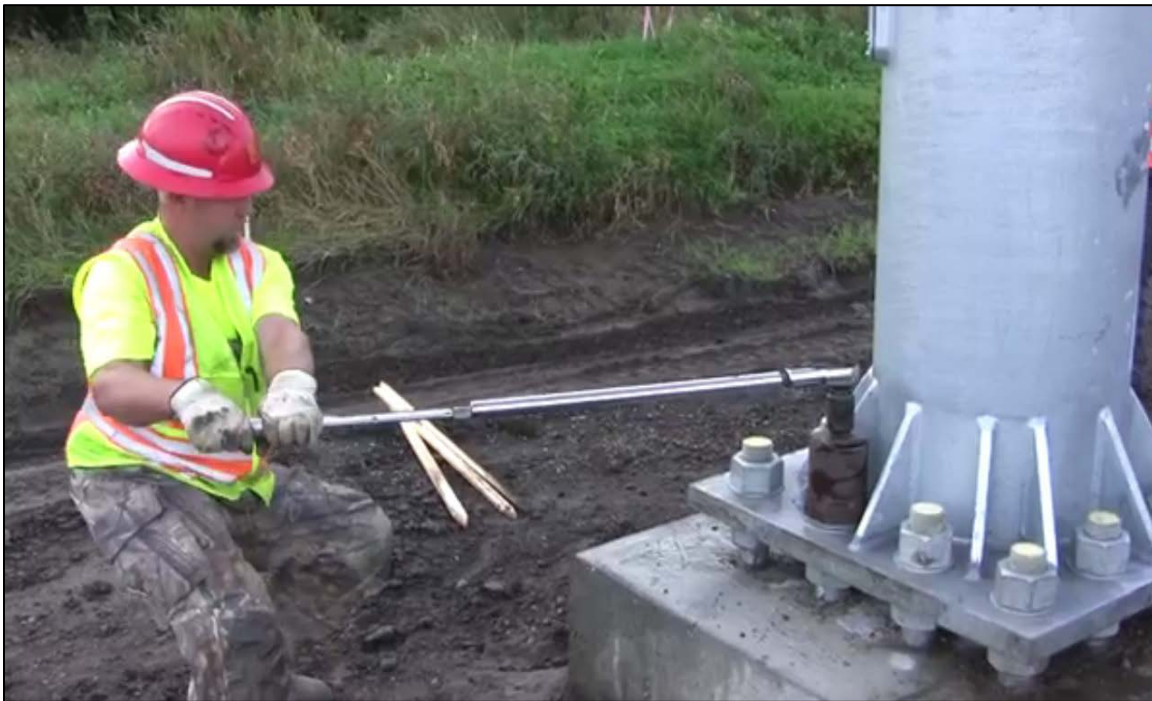
Figure 1.14 - Top Nut Tightening with Calibrated Wrench in Minnesota
