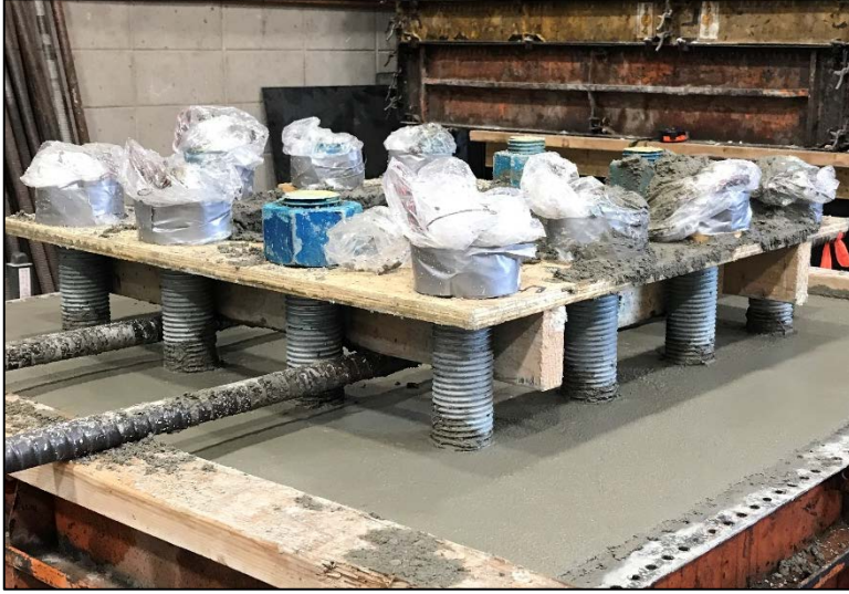
Figure 3.30 - Anchor Bolts during Concrete Curing
