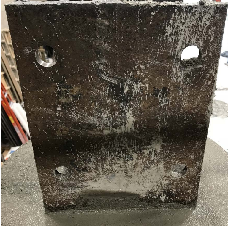
Figure 3.34 - HP10x57 Curing in Concrete
