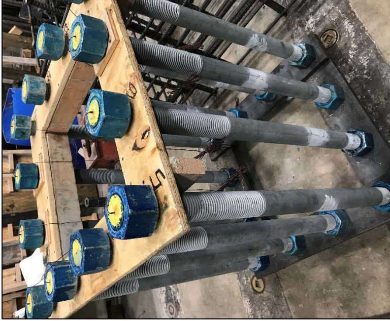
Figure 3.28 - Anchor Bolt Cage
