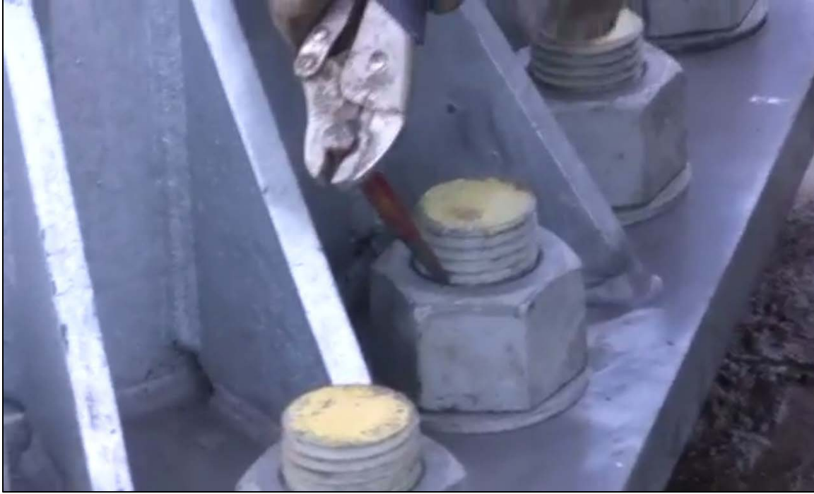
Figure 1.15 - Puncturing of Threads after Tightening
