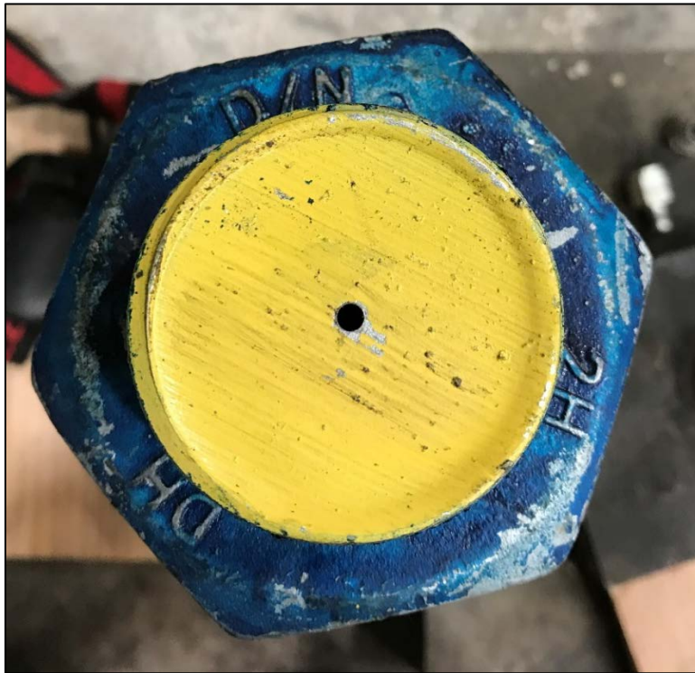
Figure 3.5 - Predrilled Hole in 2-1/4" Anchors
