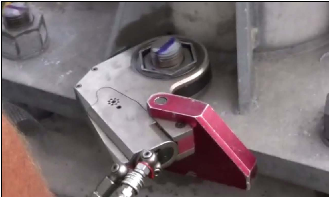
Figure 1.20 - Hydraulic Wrench Used for Maintenance Retightening
