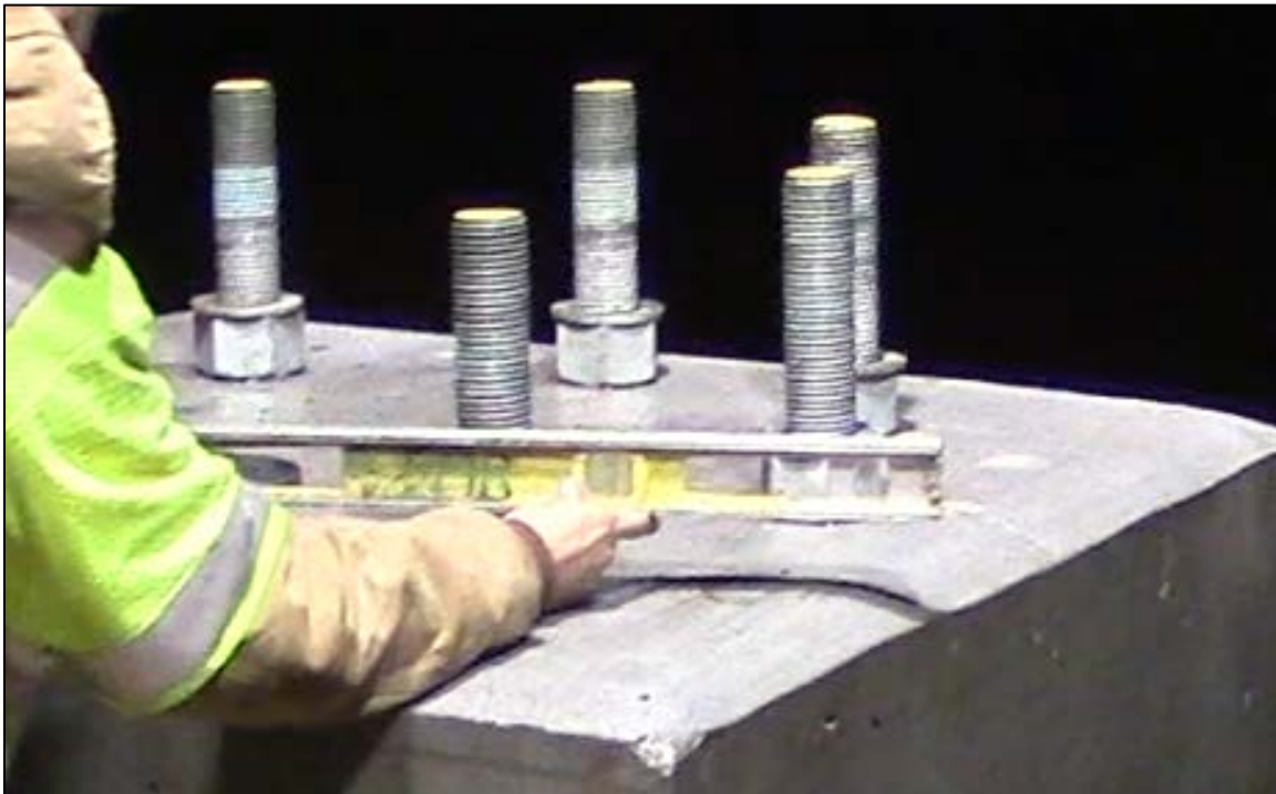
Figure 1.24 - Preparing for Pole Installation
