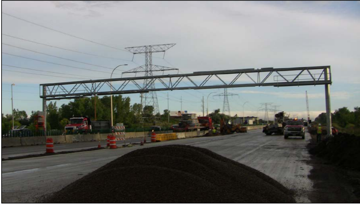
Figure 1.9 - Overhead Sign Truss on Interstate 494 Near Maple Grove
