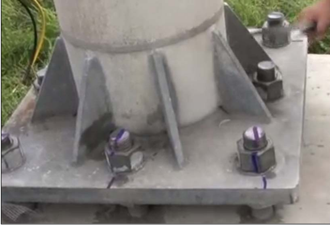
Figure 1.21 - After Maintenance Retightening
